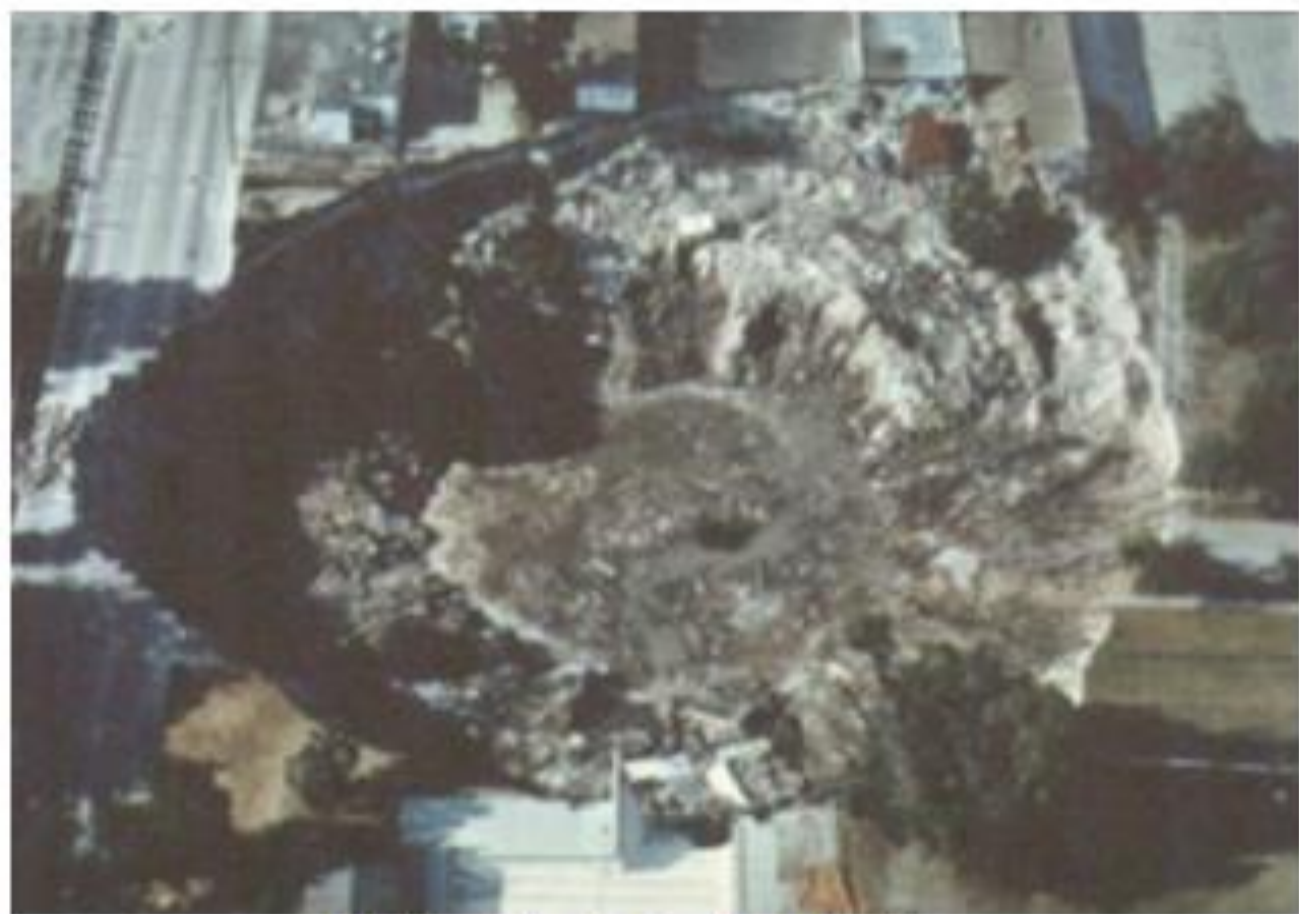
Sinkhole in Orlando, Florida
