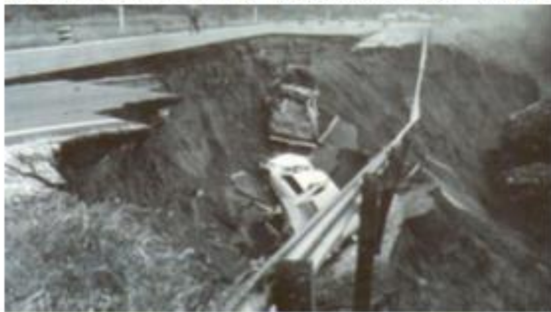
Highway Slope Failure
